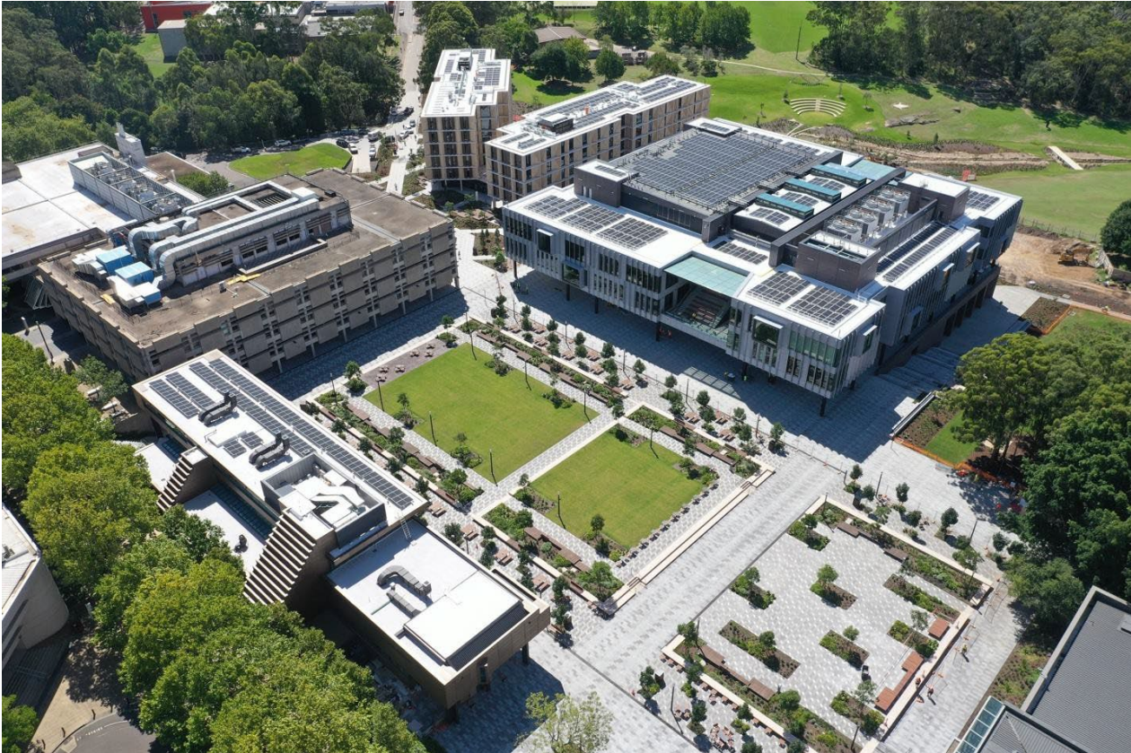
Image 2: MUCCP Central Courtyard Precinct
