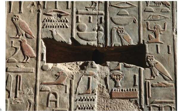
Fig. 7. Deir el-Bahari, temple of Hatshepsut, architectural elements: dovetail cramp: a) wooden original, b) stone socket (Phot. J. Iwaszczuk).
